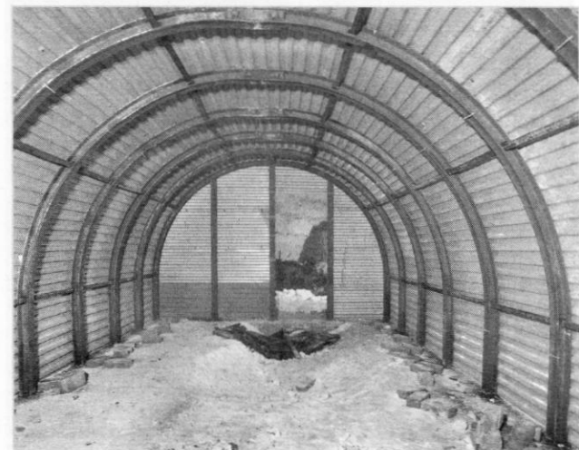
This picture shows the inside of one of the Nissan huts. The steel work is still in very good condition considering that it is approximately 65 years old.
